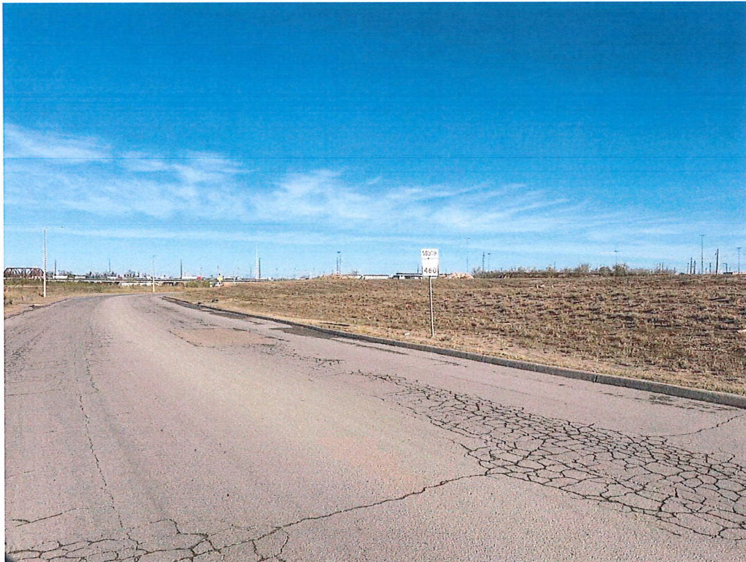
View from Industrial Blvd
