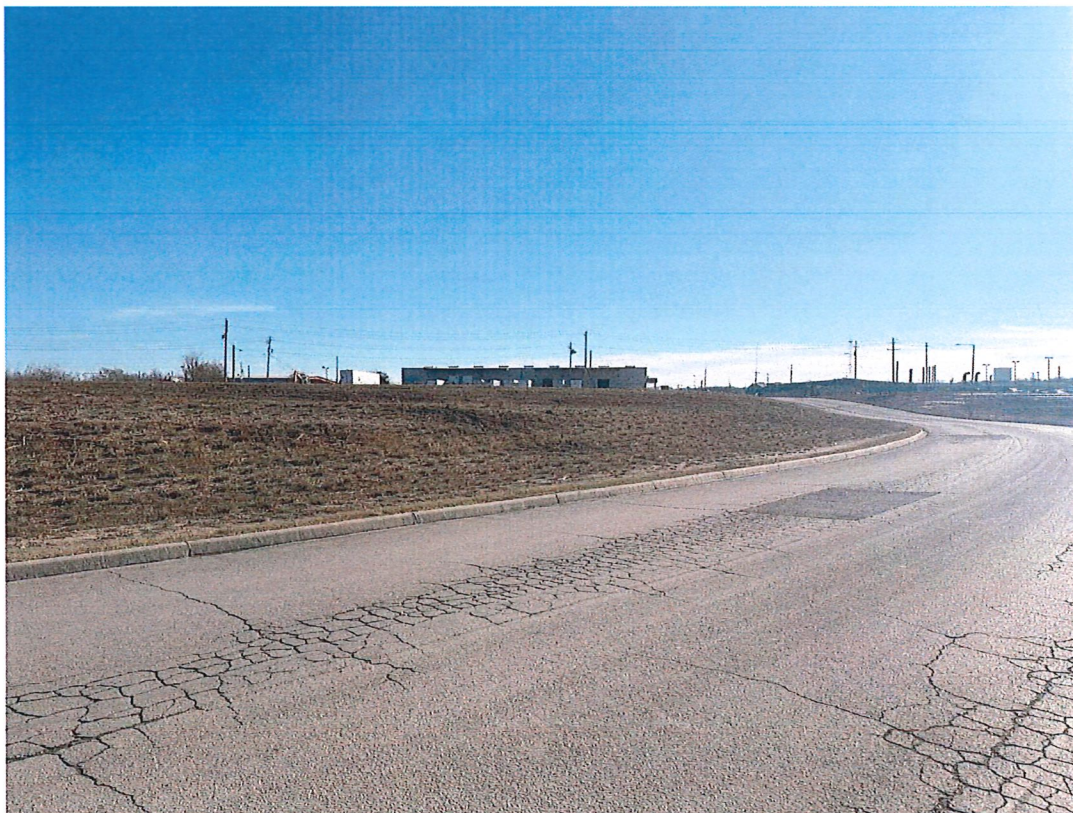
View from Industrial Blvd
