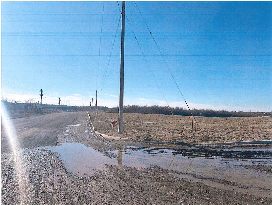
View from Industrial Spur 2 towards Industrial Blvd
