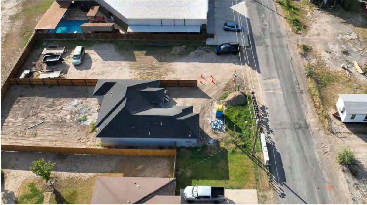
Figure 5. View from the East, showing High Noon with no curb, no sidewalk.
