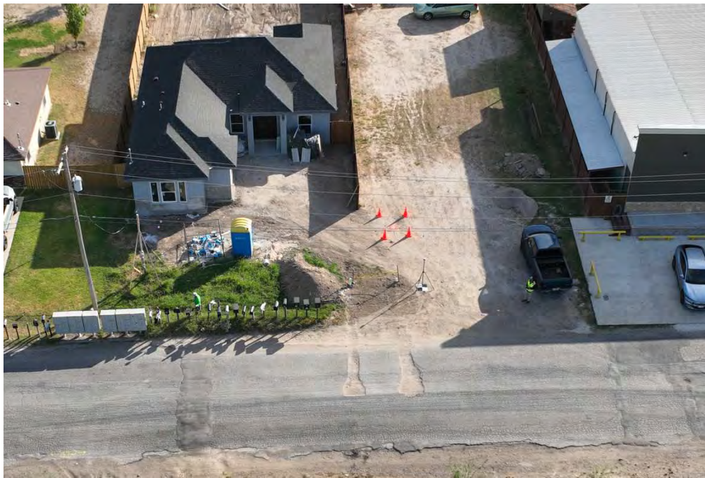
Figure 4. Drone image from the North, showing location of the two Cleanouts serving lots and a water meter for lot 2A
