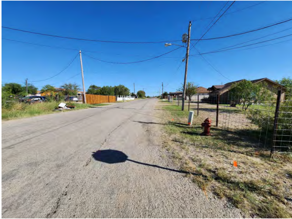
Figure 7. North corner of the property, Fire Hydrant located within the ROW
