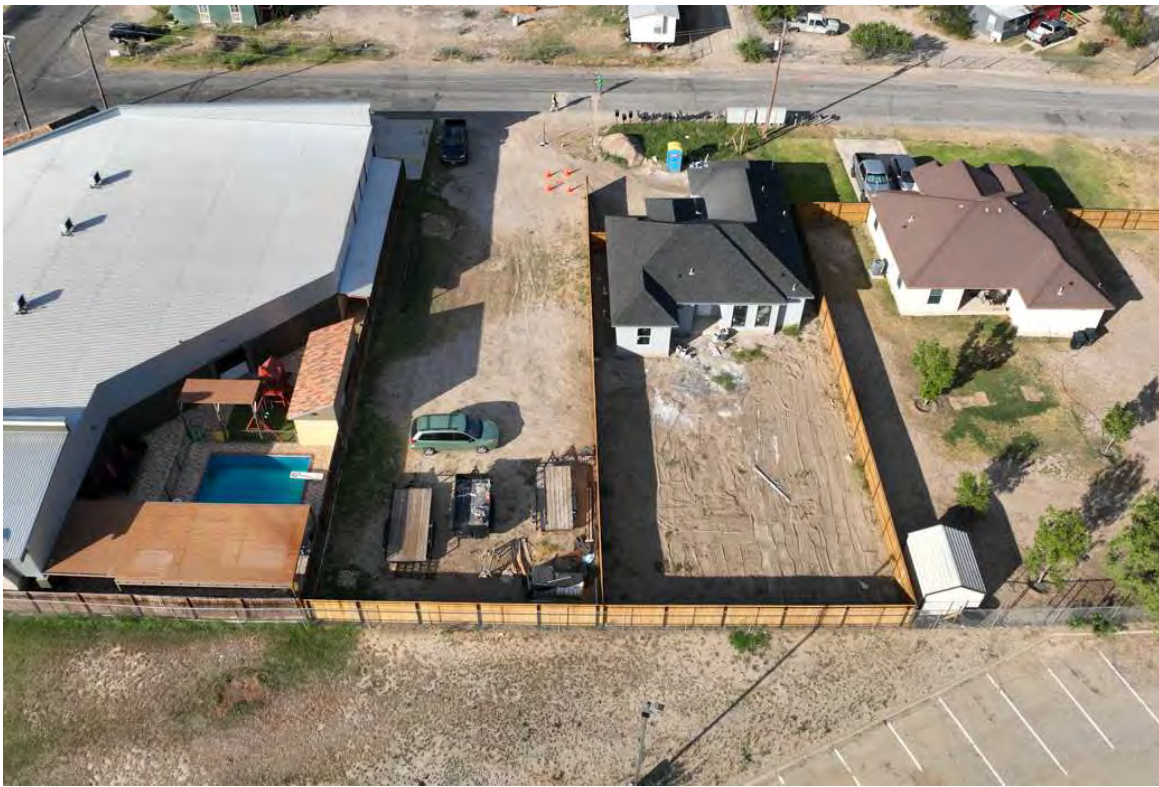
Figure 6. View from the South.
