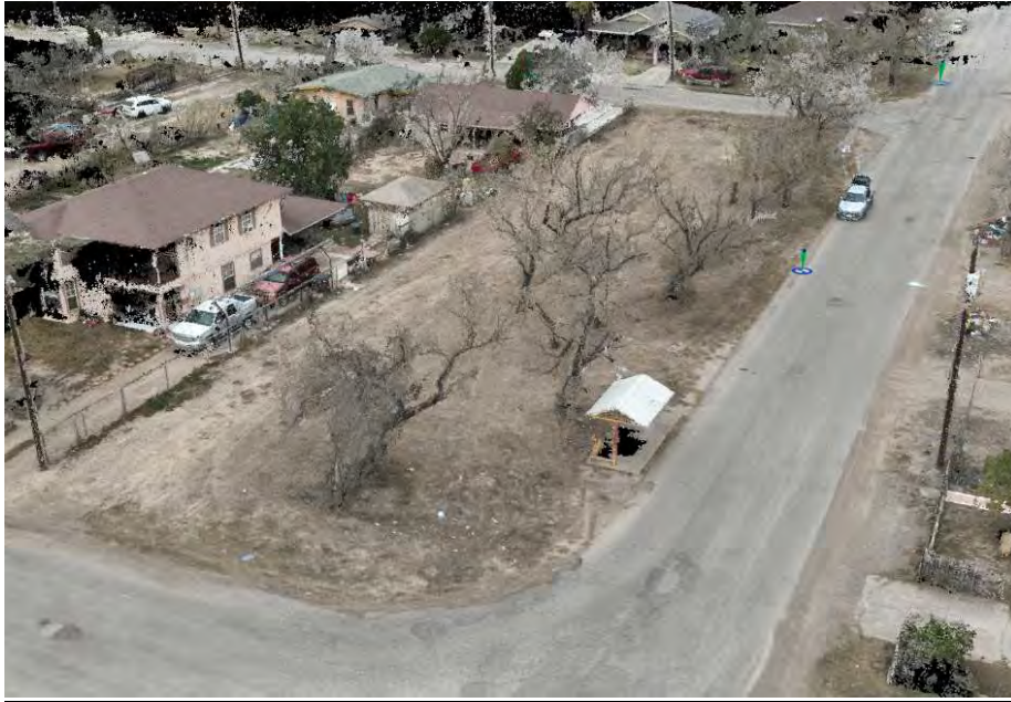
Figure 3. View from the Southeast corner of the property, (3d Point Cloud) Intersection of La Herradura Road and Erika Street
