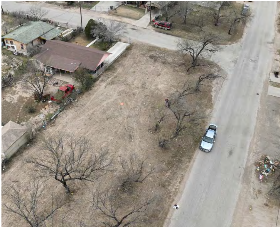
Figure 4. Intersection of Mariza street and La Herradura road, no curb and no sidewalks on the subdivision.
