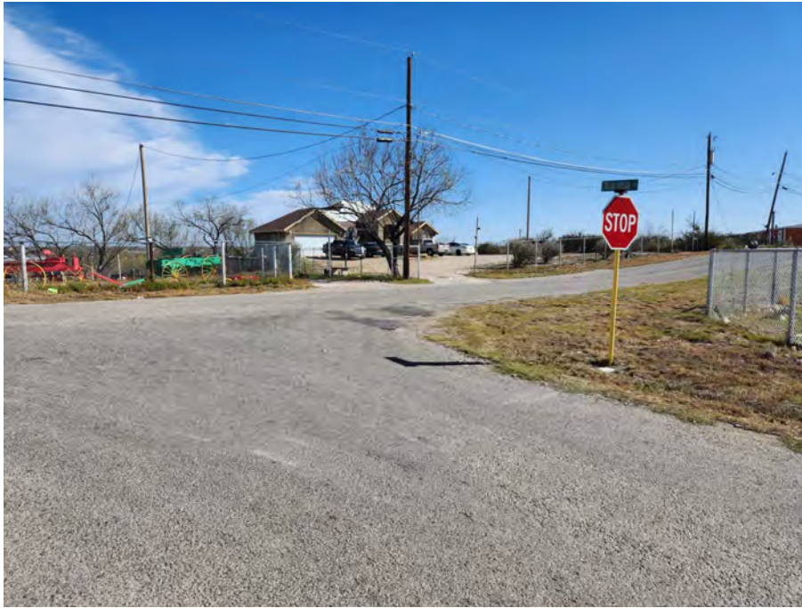
Figure 4. Intersection of Linda Vista and Chucho Dr, no curb and no sidewalks on the subdivision.
