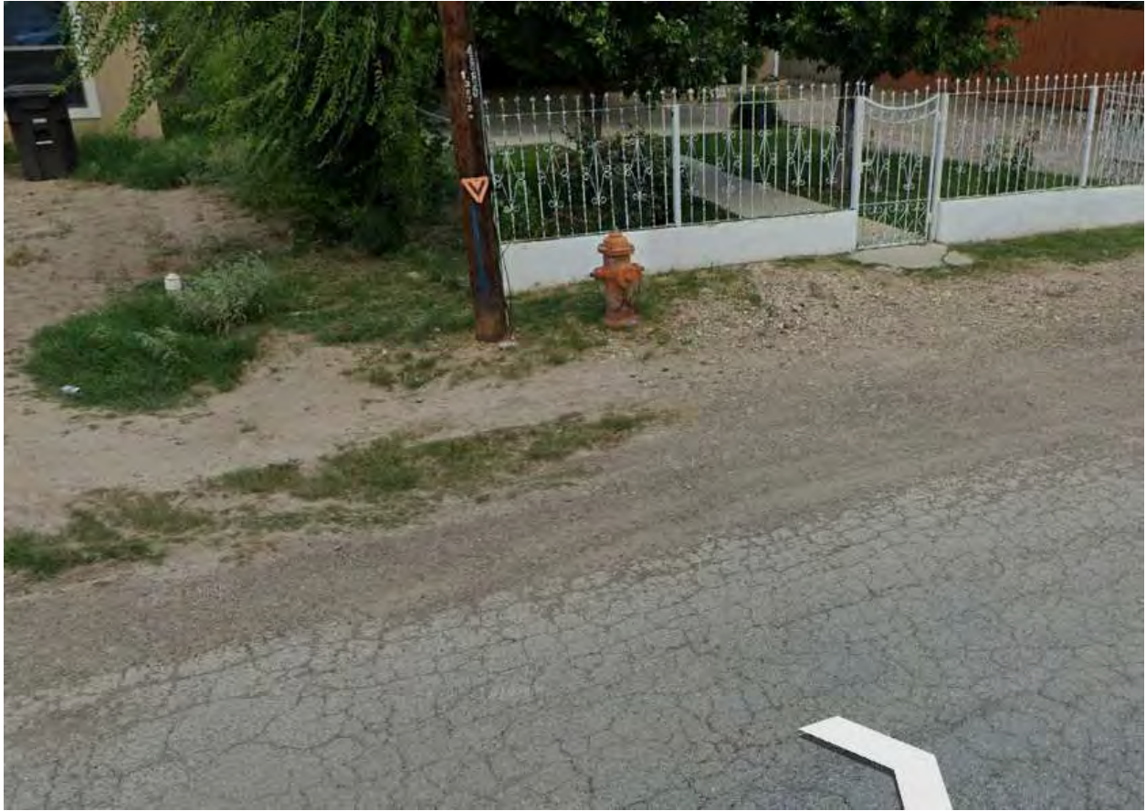
Figure 10. Fire Hydrant located across La Herradura road, on the southeast corner of the property
