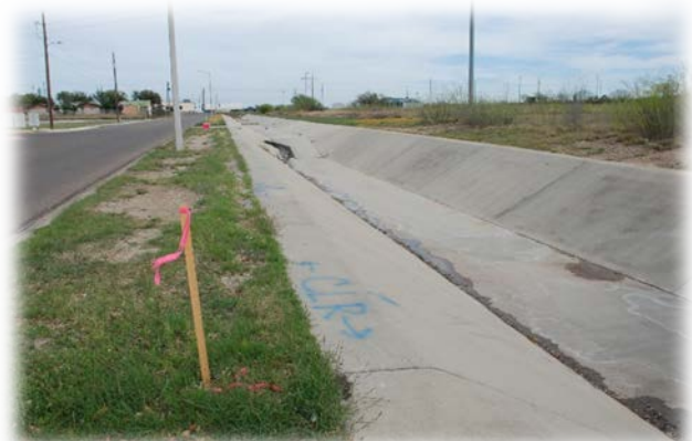
Existing concrete lined channel at Royal Ridge.
