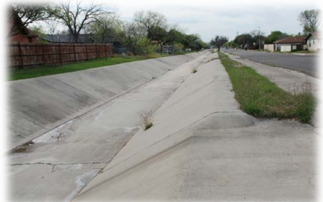
Existing concrete lined channel
