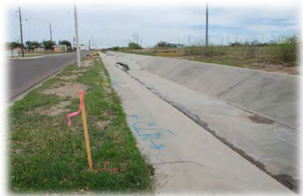
Existing concrete lined channel
