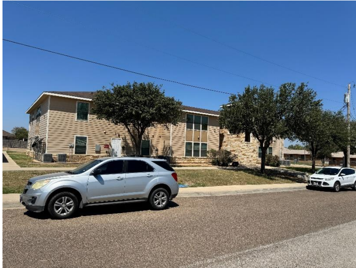
View from Basswood Street
