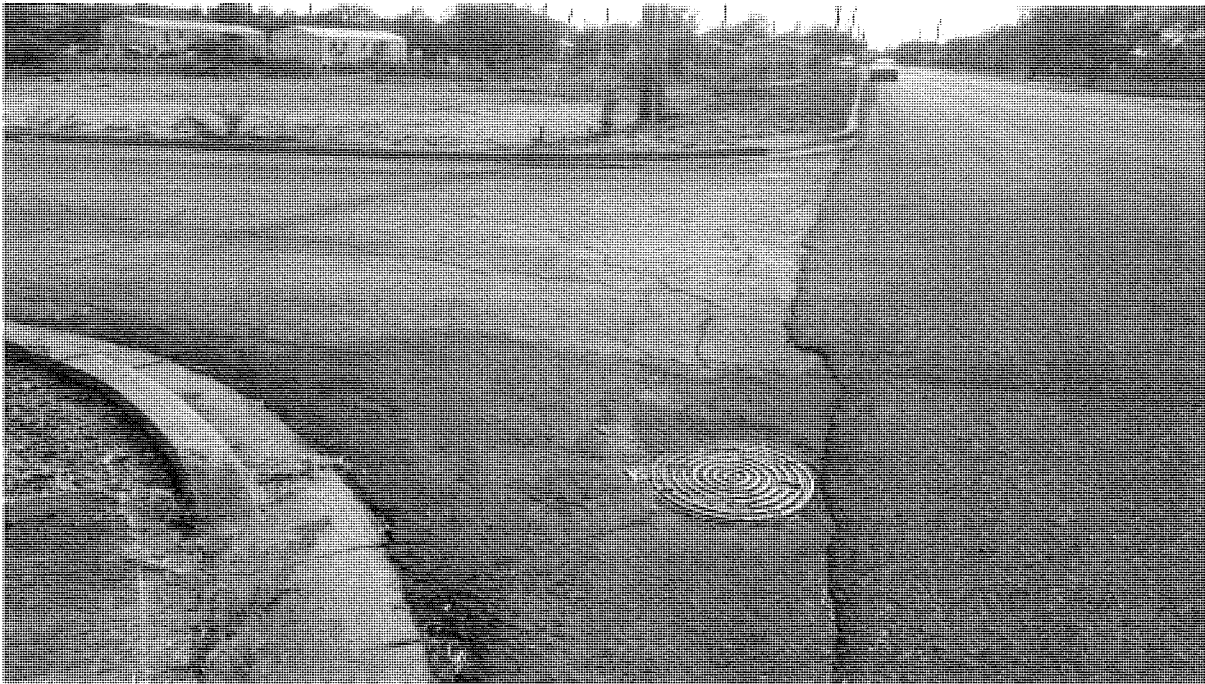
Figure 7. Intersection of Doctor Gates street and Chavarria/Becos street, northeast corner of the property
