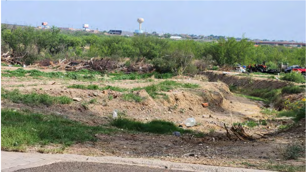
Figure 5. Existing drainage way located to the west of the property.
