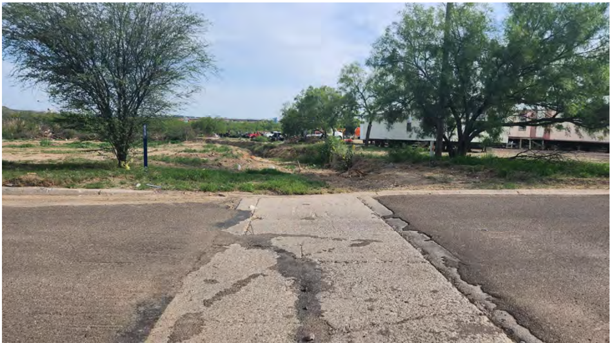
Figure 4. Existing drainage way located to the west of the property.
