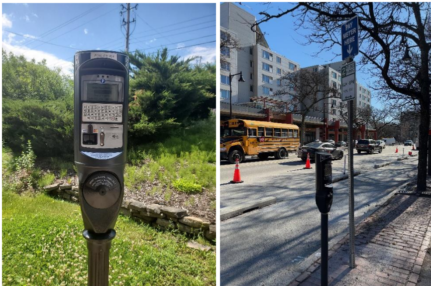
Figure 11 - mkORA Lite pay-by-plate pay stations installed on street
